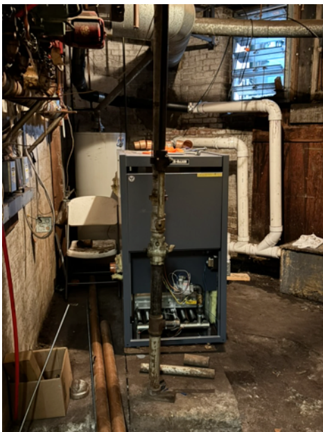
Work is continuing on our replacement furnace for the Parish House. Here you can see the “knock-down” furnace in last week’s photograph has been assembled and the plumbing is now being installed.
