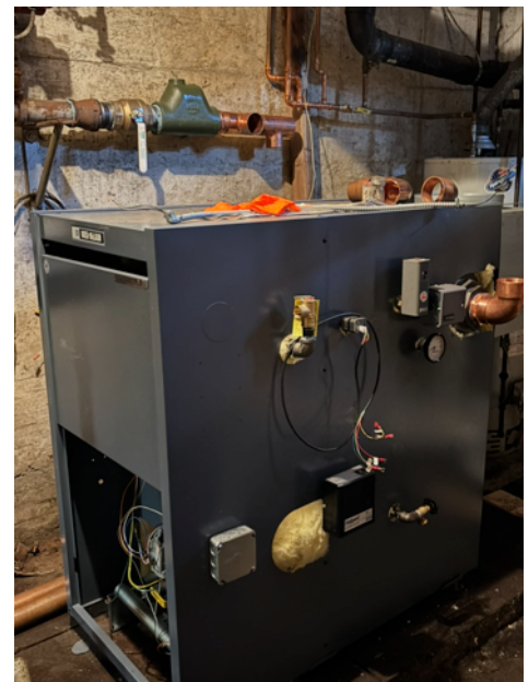
Work is continuing on our replacement furnace for the Parish House. Here you can see the “knock-down” furnace in last week’s photograph has been assembled and the plumbing is now being installed.
